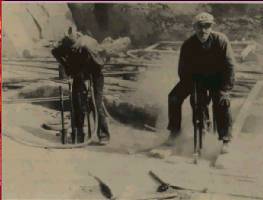
FIGURE 12. Jackhammer drilling without dust control. (About 1936.)
