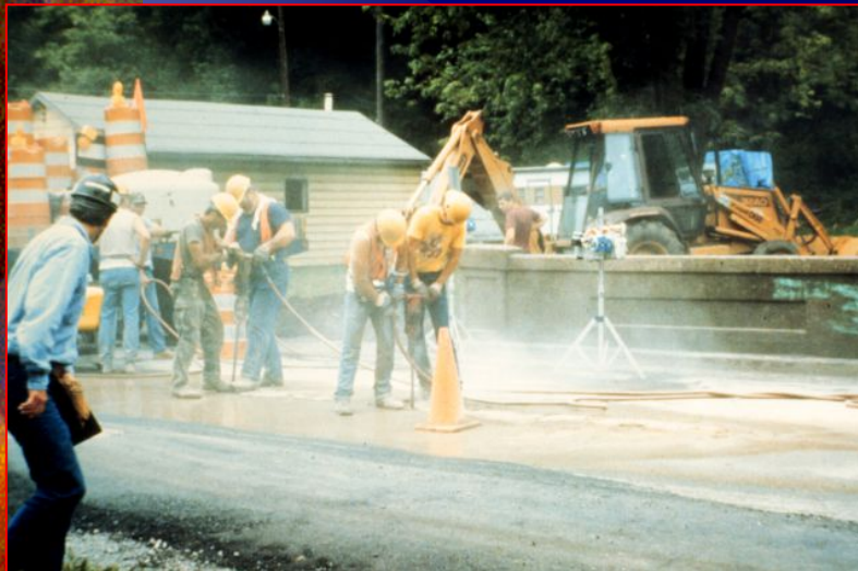
FIGURE 12. Jackhammer drilling without dust control. (About 1936.)
