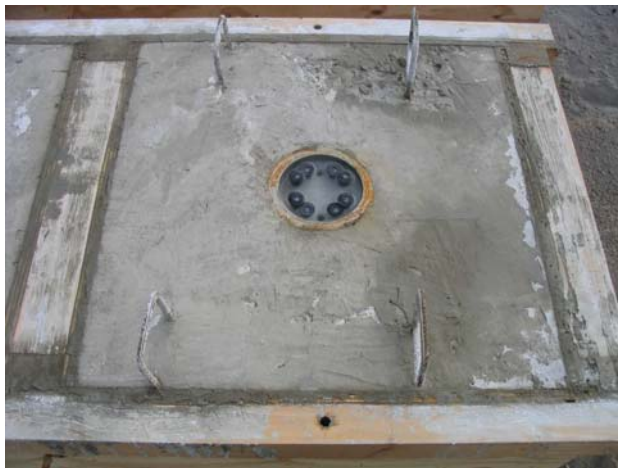
Figure 6b: Embedded intermediate piece flush with surface of concrete block
