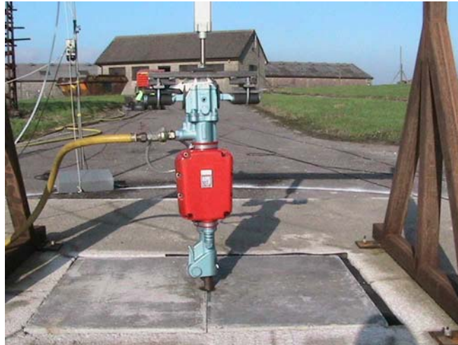
Figure 3b: Both parts of screening slab fitted over concrete block
