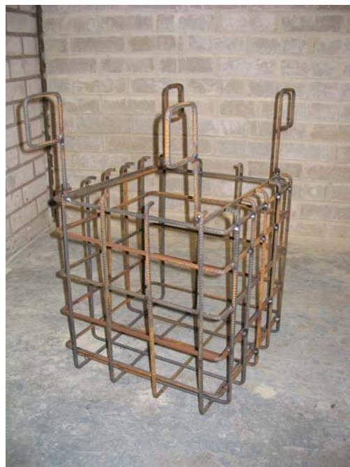
Figure 4: Lightly tied reinforcing steel rods
