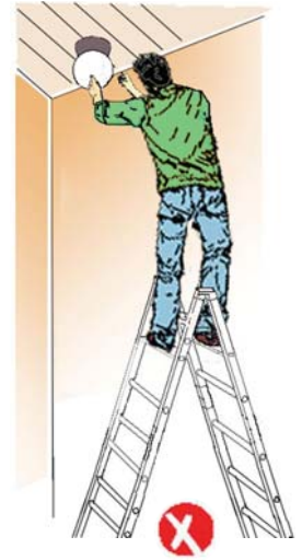
Figure 3 - never straddle a stepladder
