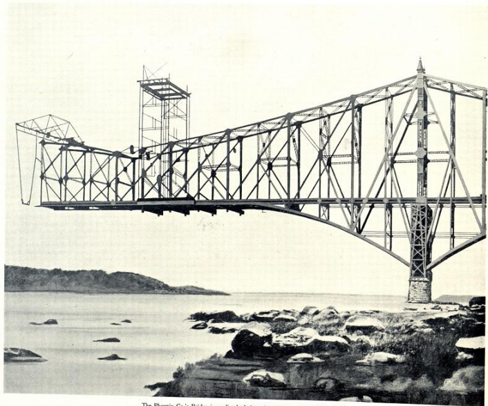
The Phoenix Co.'s Bridge immediately before the collapse, August 29th, 1907
