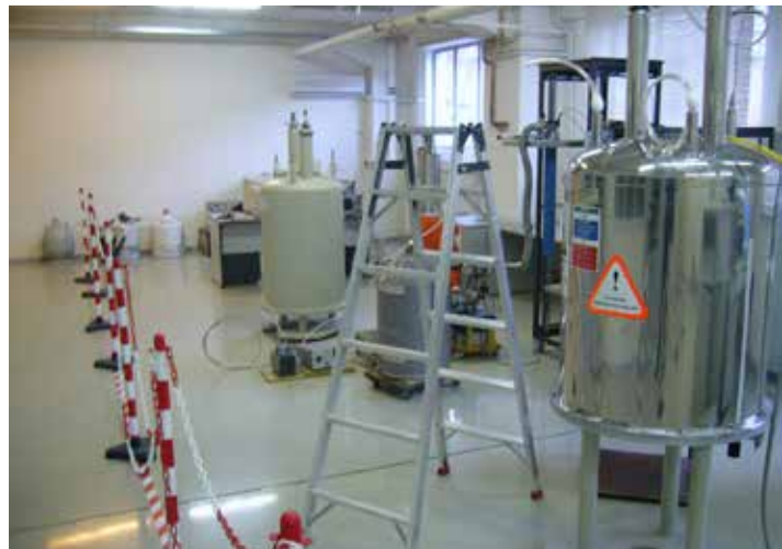
Figure 2.4 — Demarcation of the restricted area by a chain-link barrier and marking the floor
