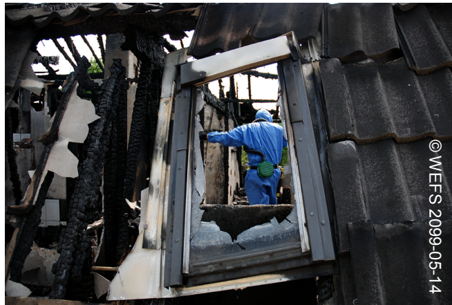
Asbestos removal work after a fire
