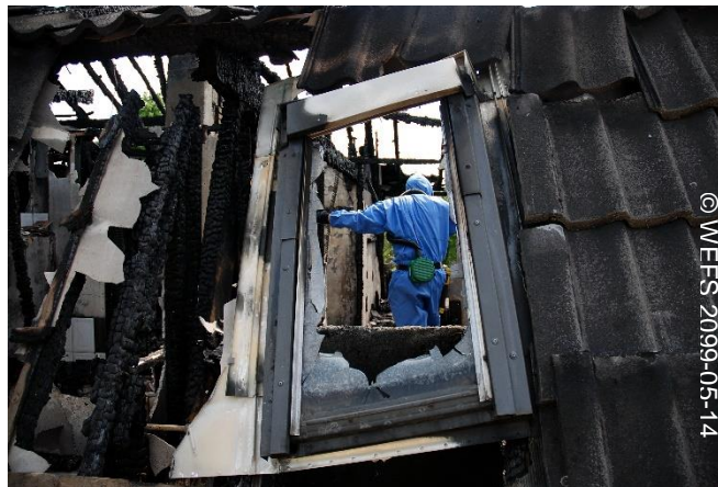
Asbestos removal work after a fire
