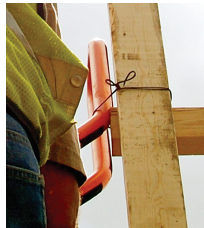
PHOTO COURTESY OF KIEWIT POWER CONSTRUCTORS
