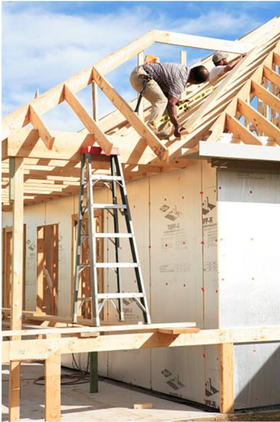
Image 870: OSHA Training Institute, Southwest Education Center http://www.elcosh.org
