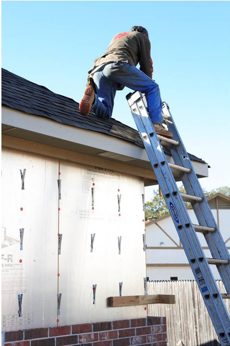
Image 891: OSHA Training Institute, Southwest Education Center http://www.elcosh.org
