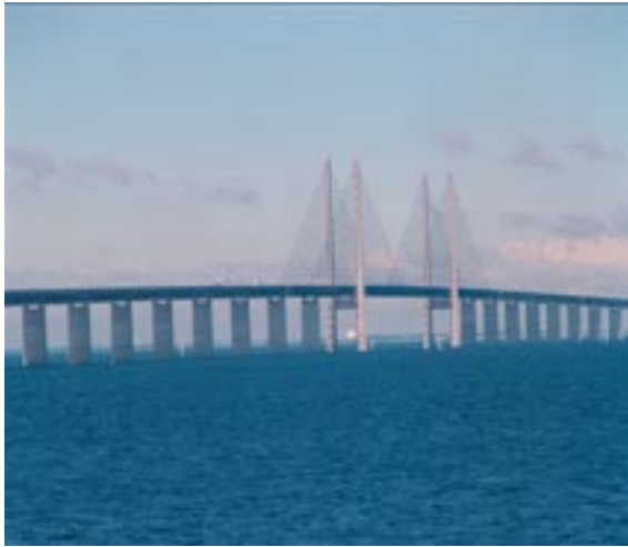
Figure 12: The Oresund bridge
