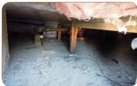
Exterior entrance and crawl space
