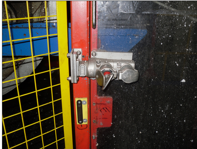
Figure 4 Example of an interlocked guard with trapped key
