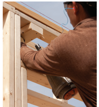
Nail penetration through the lumber is a special concern where the piece is held in place by hand
