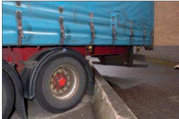
Figure 7 Concrete wheel stop
