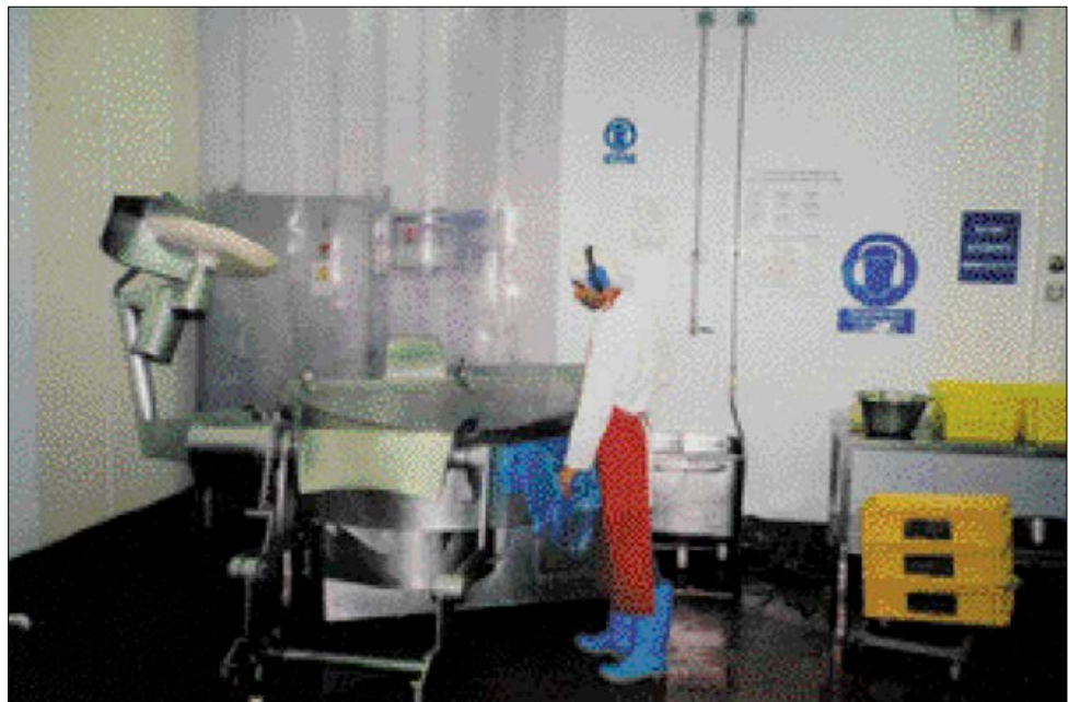
Solution: bowl chopper and mincer in isolated area away from main production area
