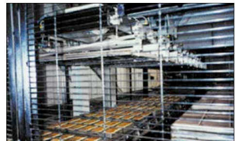
Solution: new robot installed for lidding/de-lidding tins
