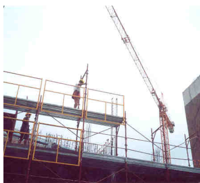
posa telai verticali
