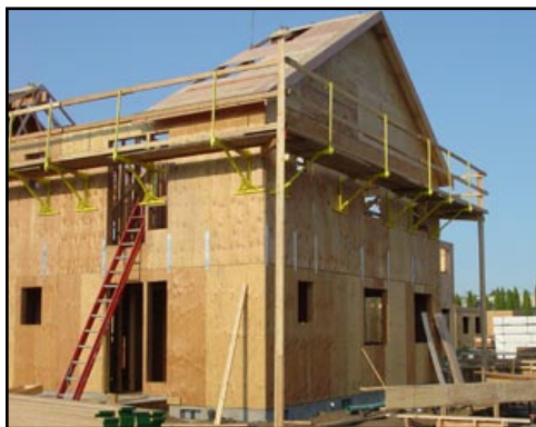
Manufactured exterior carpenter's bracket scaffolding.
