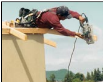
Hip rafter plumb cut: Is there a safer way to do this?
