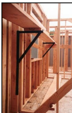
Interior scaffold brackets designed by the home builder.
