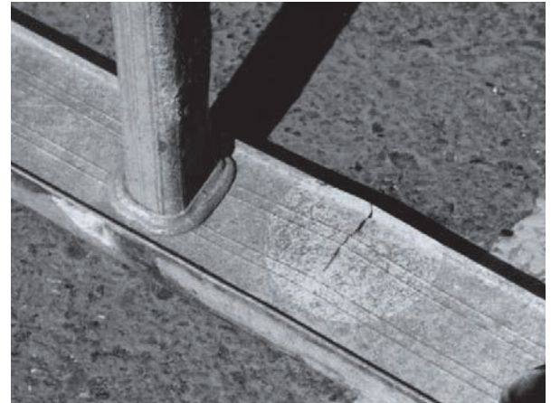
Equipment inspections are critical. Do you see the small fracture in this picture?
