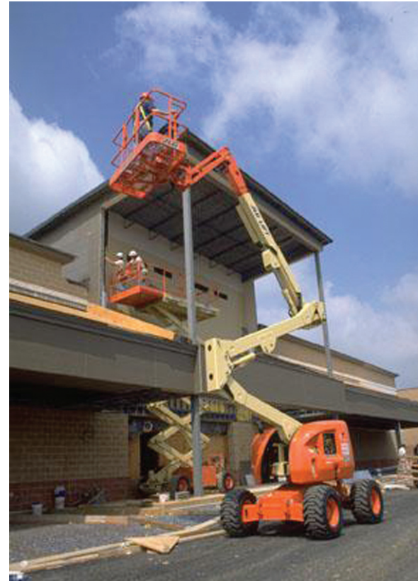
If you work from an aerial lift, you must be protected from falling.
