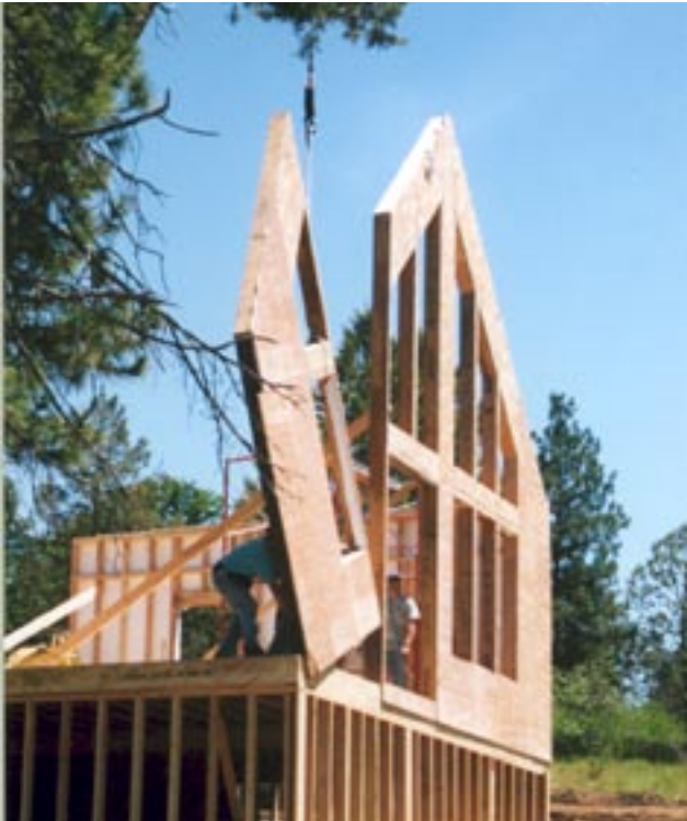
Photo credit: Integrated Building Solutions of Oregon
