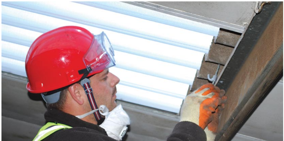
Securing fixings to newly installed sheet
