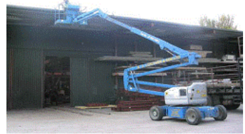
Using a MEWP to clean a gutter
