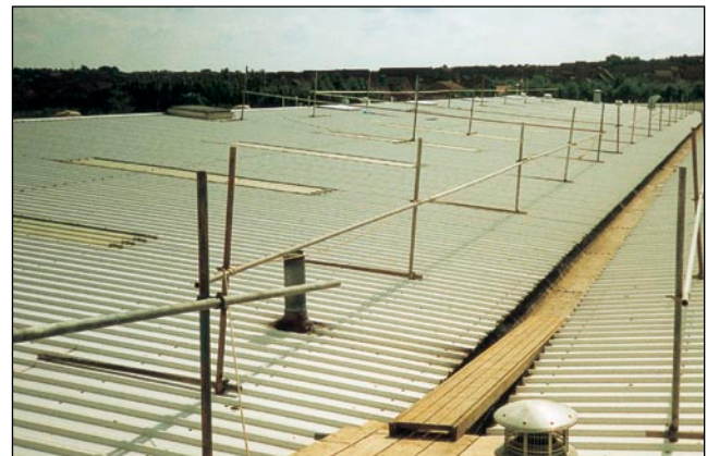
Figure 21 Demarcation barriers on a large, non-fragile roof, preventing access to the adjacent fragile roof lights. The roof lights are at least 2 m from the barrier
