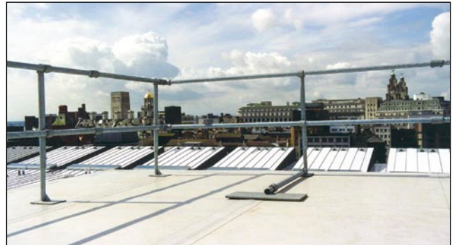
Figure 18 Temporary flat-roof edge protection. Adjustable supports enable work to progress with protection in place (Image courtesy of Safesite Limited)
