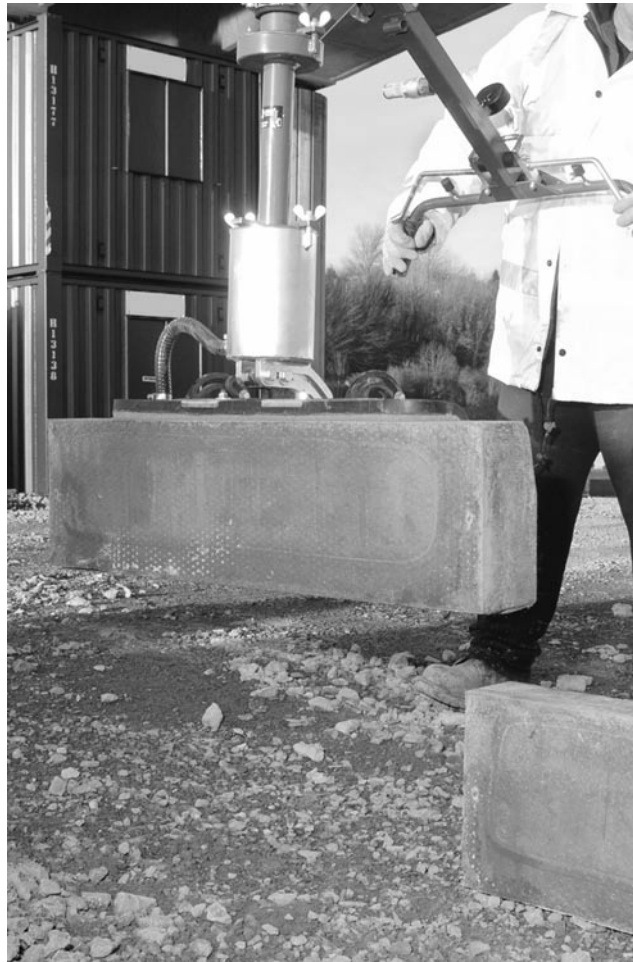
Figure 38 Handling kerbs using a vacuum lifter
