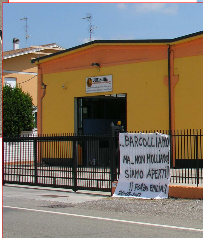
Tamponature in muratura
