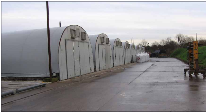
2 Typical sheds used to house racks and shelves
