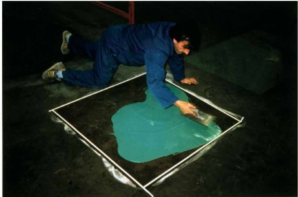
Figure 14 Damping compound being applied to metal decking
