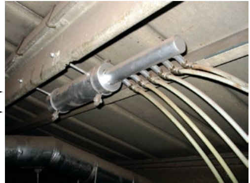
Figure 21 Multiple air exhausts piped to a manifold and silencer
