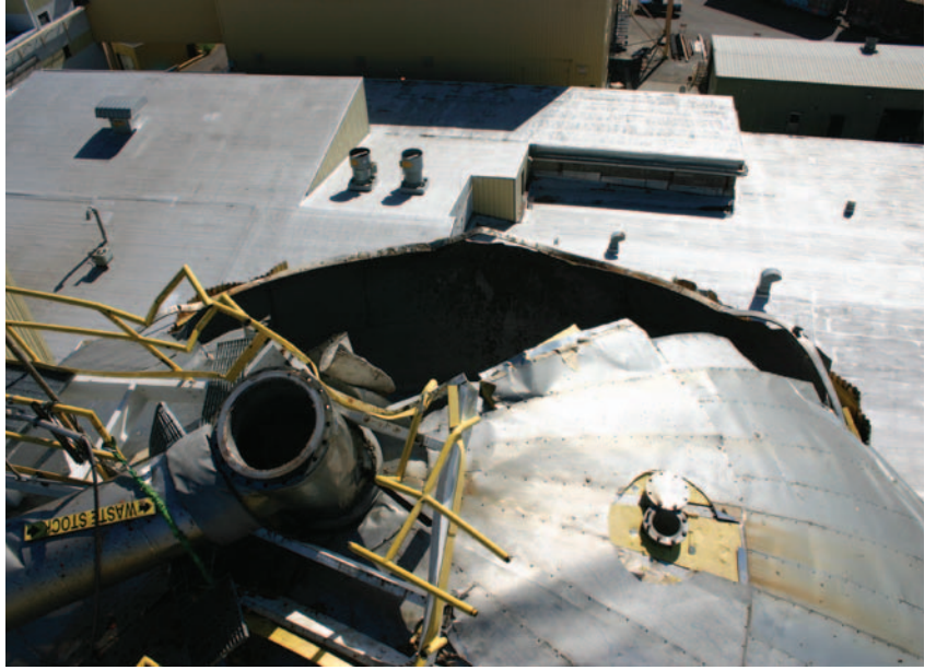
Views of the storage tank involved in the 2008 explosion at Packaging Corporation of America.
