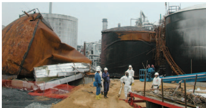
A view of the flammable storage tank involved in the accident at the Motiva Refinery.
