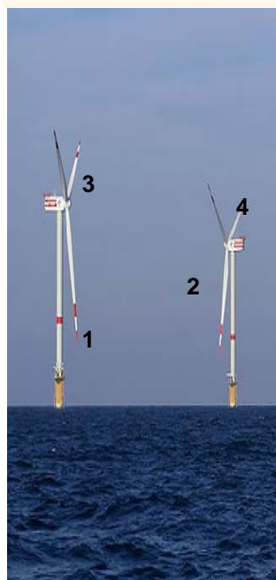
Right offshore wind turbines
