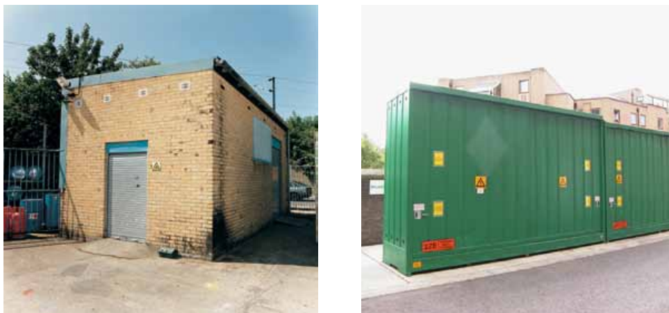
Figure 49 Flammable liquid stores should be secure and have suitable markings, ventilation and spillage retention
