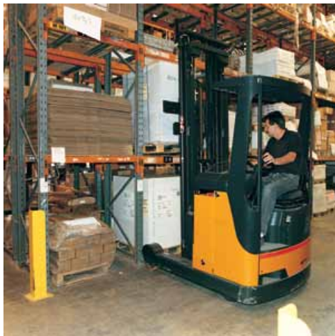
Figure 3 Racking should be securely fixed and have aisles wide enough to allow manoeuvring
