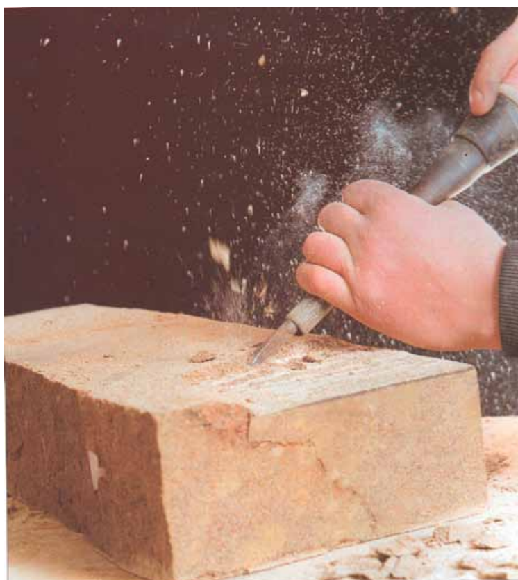
Photograph 9 Keeping stone well soaked and damp reduces release of fine stone dust particles especially for hand and pneumatic chiselling work
