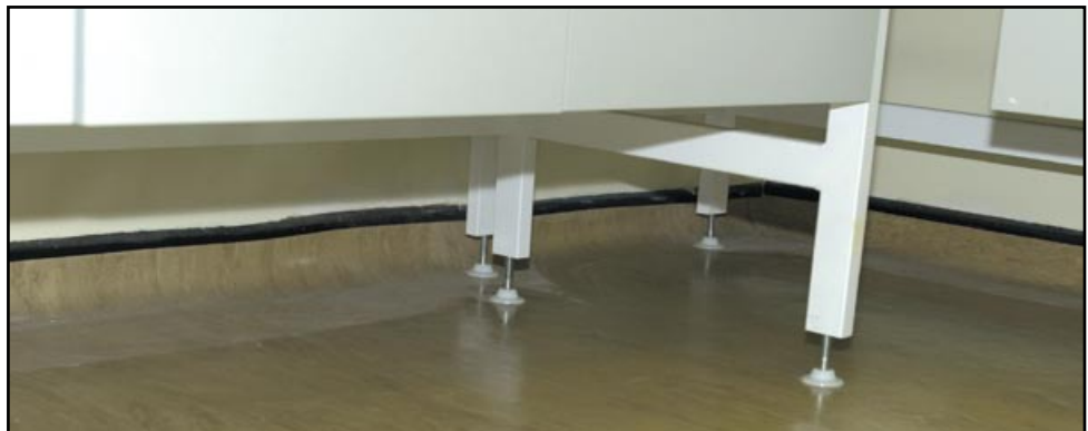
Figure 10 Floors covered to walls for easy decontamination
