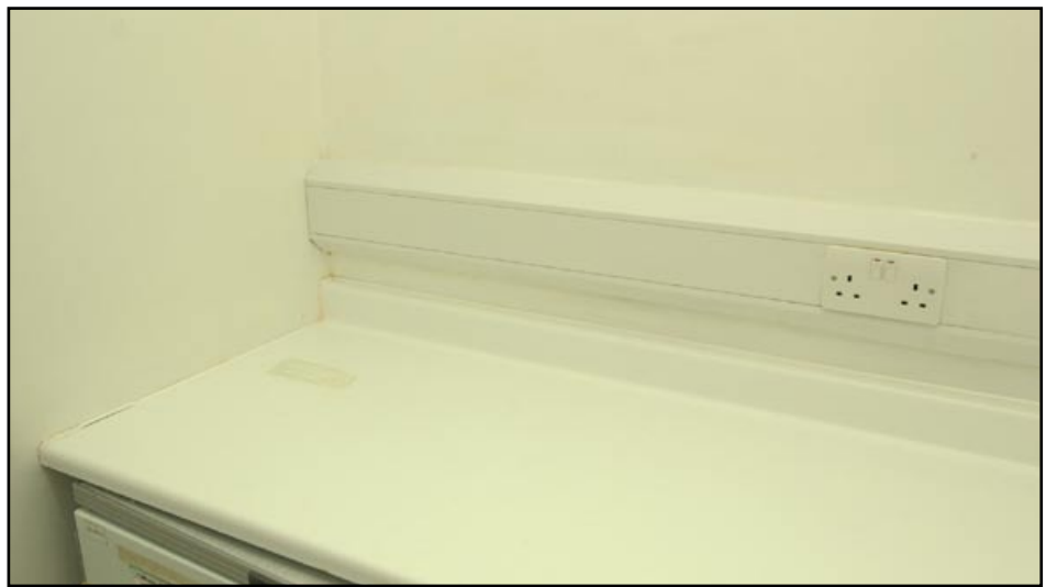
Figure 8 Bench surface sealed to wall
