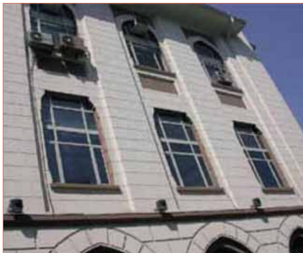
[Fig. 12] - Palazzo storico verniciato con Nanotex a Izmir, Turchia (dopo 18 mesi) / Historical building painted with Nanotext in Izmir Turkey (after 18 months)
