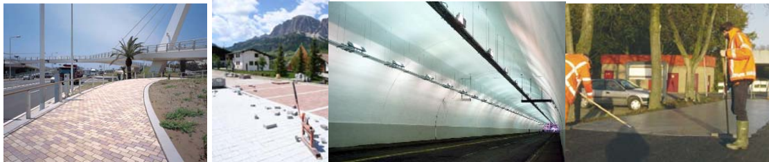
Figure 0-9 From left to right: a side walk in Japan paved with NOxer®, TX Aria road pavement blocks and tunnel coating (Italcementi), a KonwéClear road ( Bouwend Nederland Podium 22 , 14 Dec. 2006).
