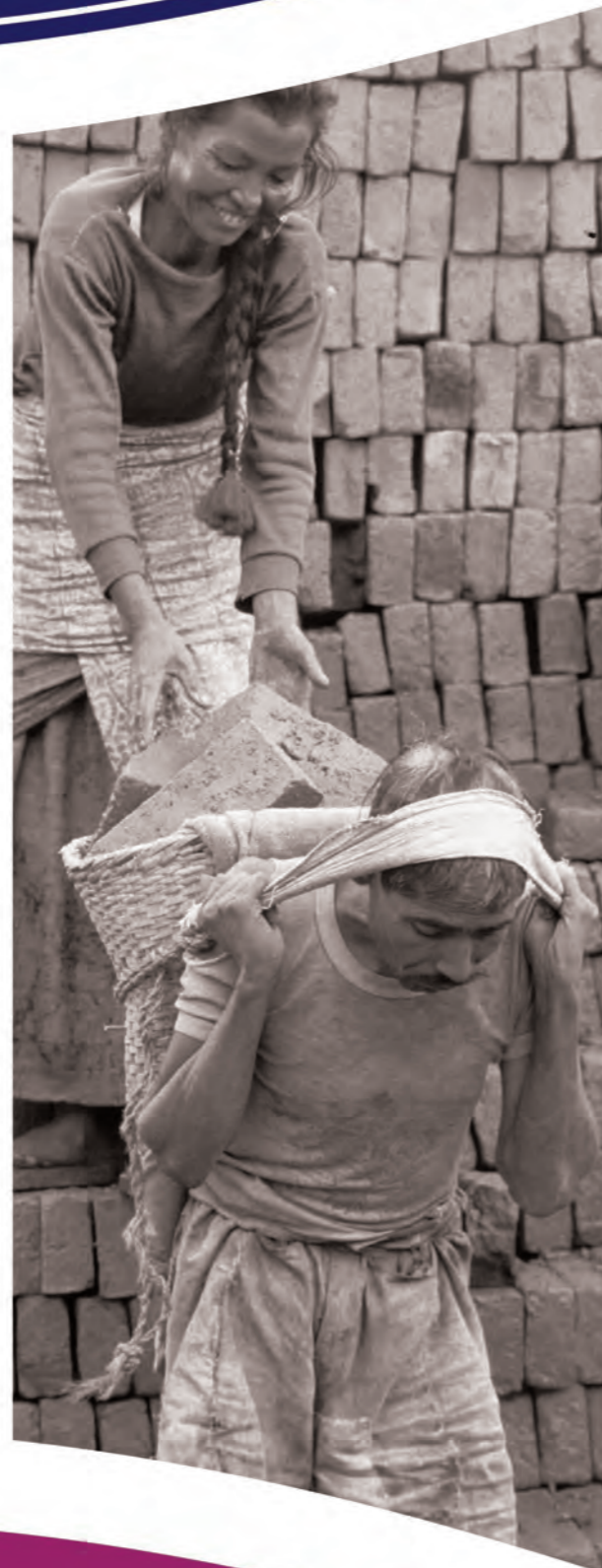
IMAGE, RIGHT Man and woman working in construction, Nepal © ILO
